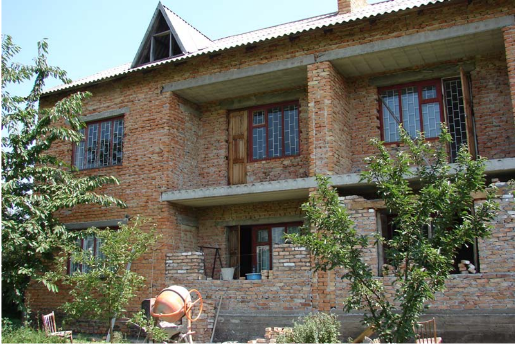
Renovations are now underway
