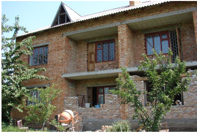
Renovations are progressing (new pictures soon)
